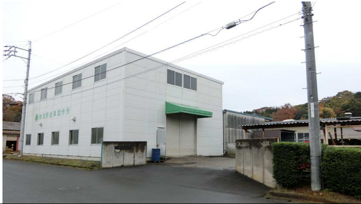
Head Office: Processing of parts and assembling
